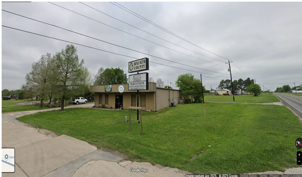
Corner View of JP2 Building. HWY 75 N is on the right side in picture.
