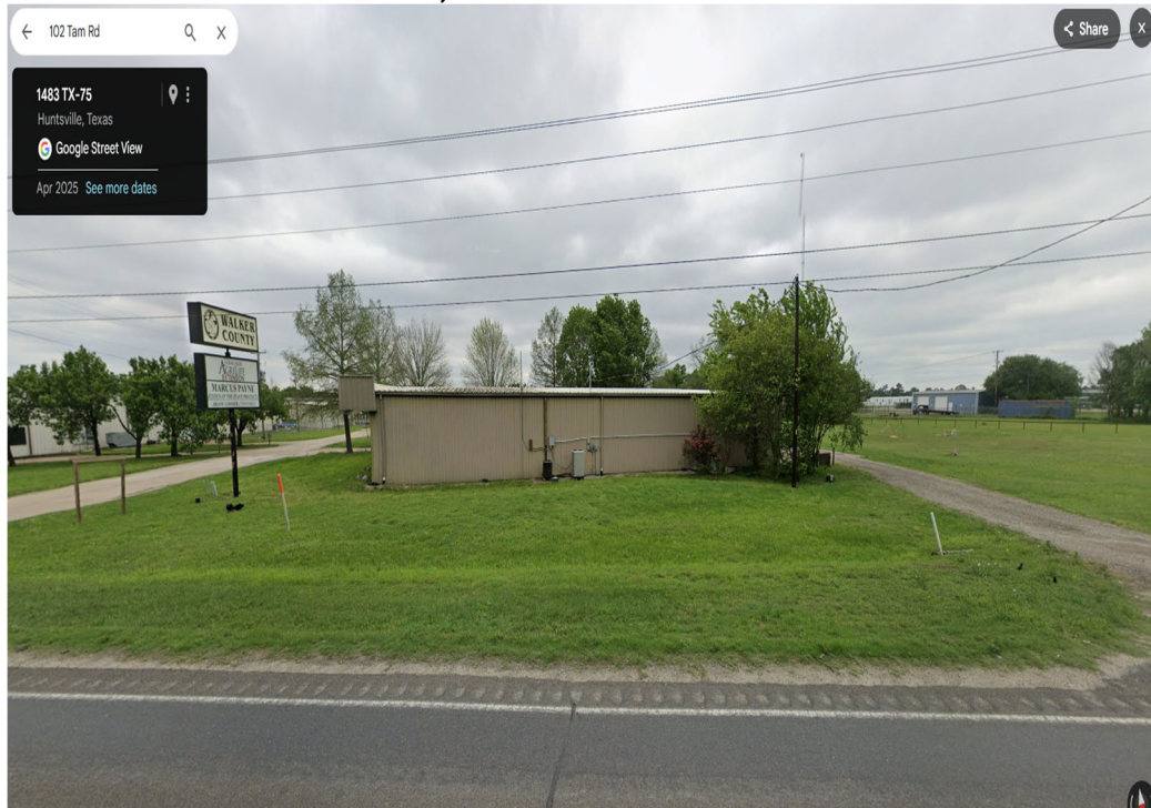
Side View of JP2 Building (HWY 75 N)- Preferred side of Generator Installation.
