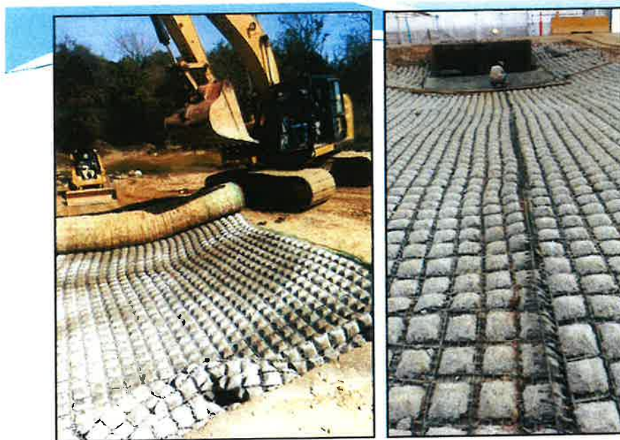
Figure 2: Flexamat Plus During Construction Being Rolled and Tied per Specifications
