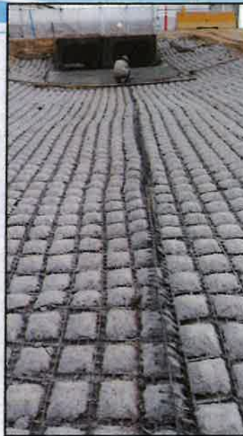
Figure 2: Flexamat Plus During Construction Being Rolled and Tied per Specifications
