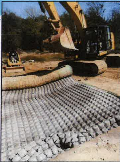
Figure 2: Flexamat Plus During Construction Being Rolled and Tied per Specifications
